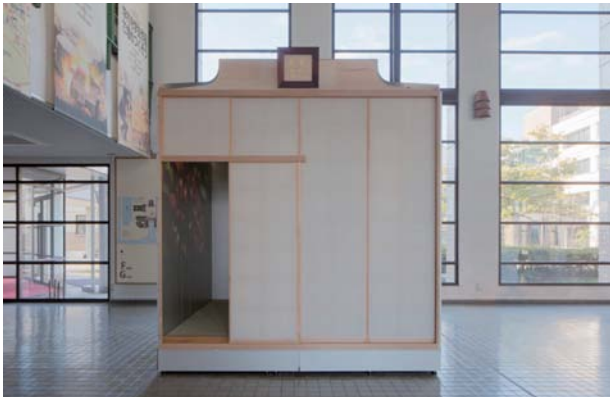
Photo 12: New timber-paper facade of the aluminum teahouse.
