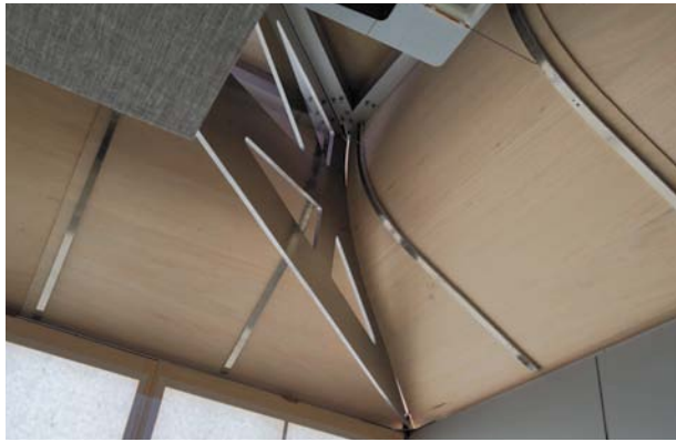
Photo 11: New roof beam
